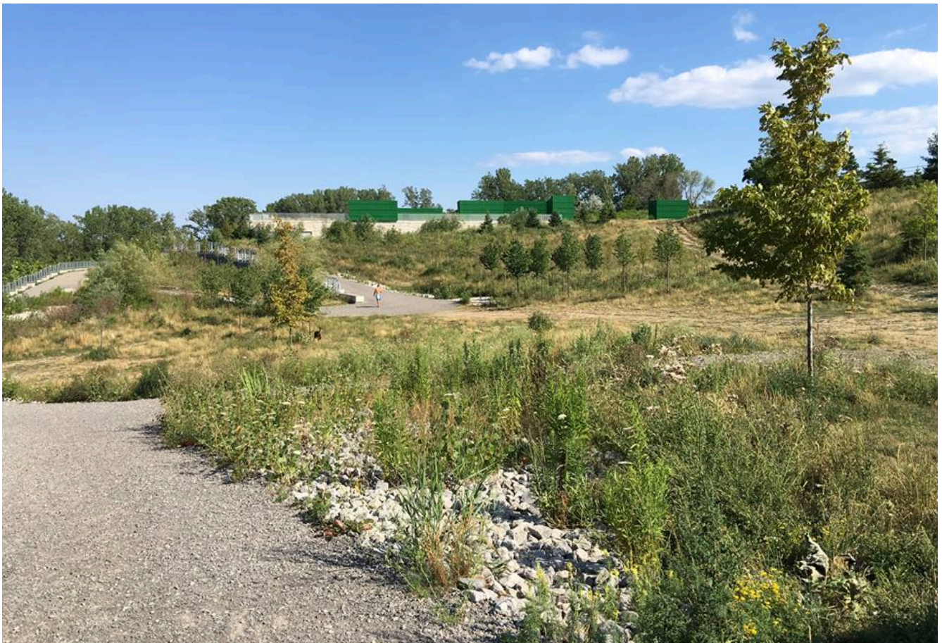
Stable slopes at Mississauga's Jack Darling Park Dog Park, built around and on top of a water treatment plant. Note the lush vegetation and thriving, unprotected trees.
