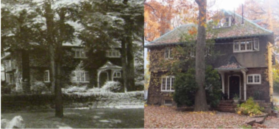
Figure 3- 72 Wells Hill Avenue (1933, left, 2012, right)
