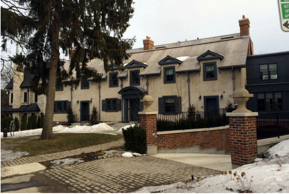
After: New additions on far left and right side of exterior, and underground garage entrance.
